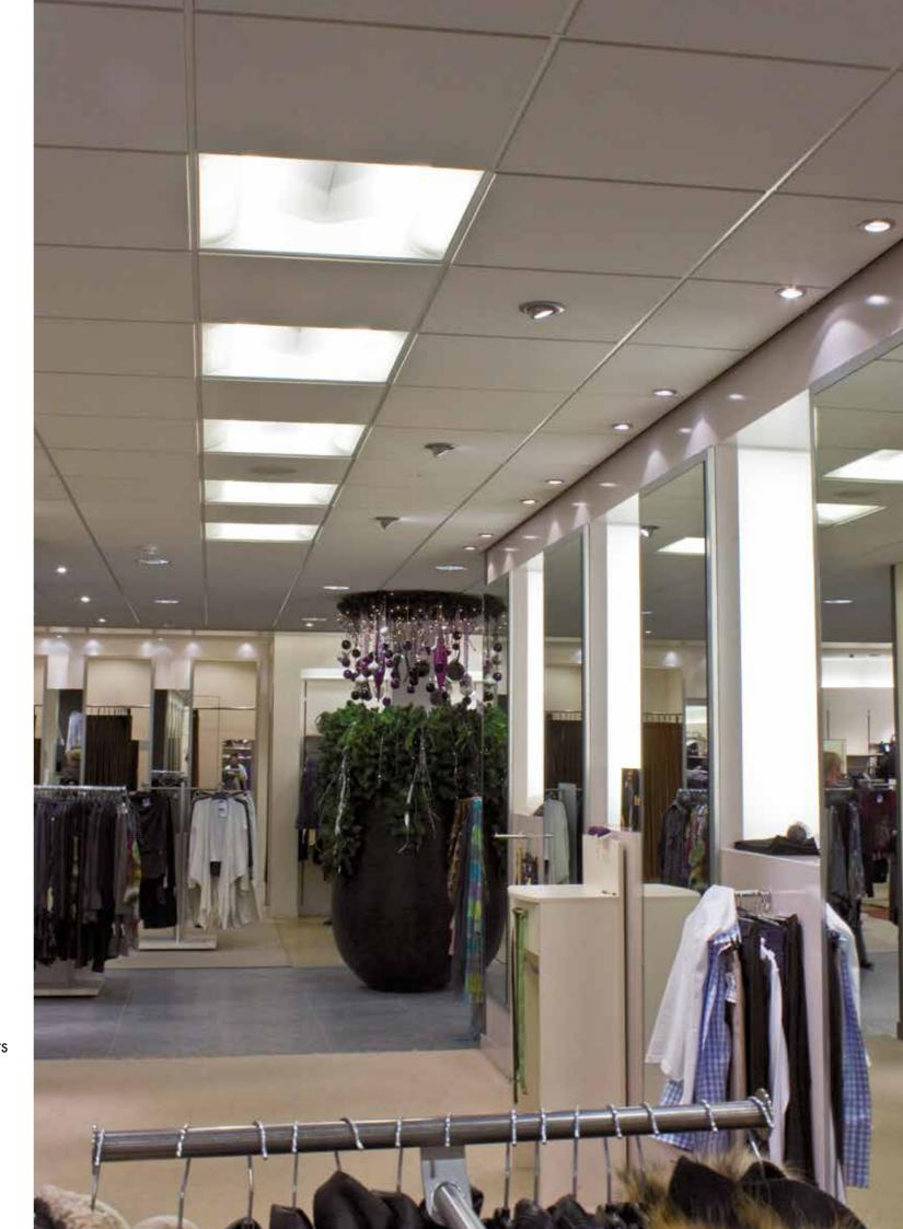
Recessed LED downlight. Body is made of steel and aluminium and it is available in all RAL colours. Light source - Philips, Osram or Tridonic LED module. Standard EVG ballast, DALI or Touch Dali version on request. Passive cooling, optional IP44 diffuser.
