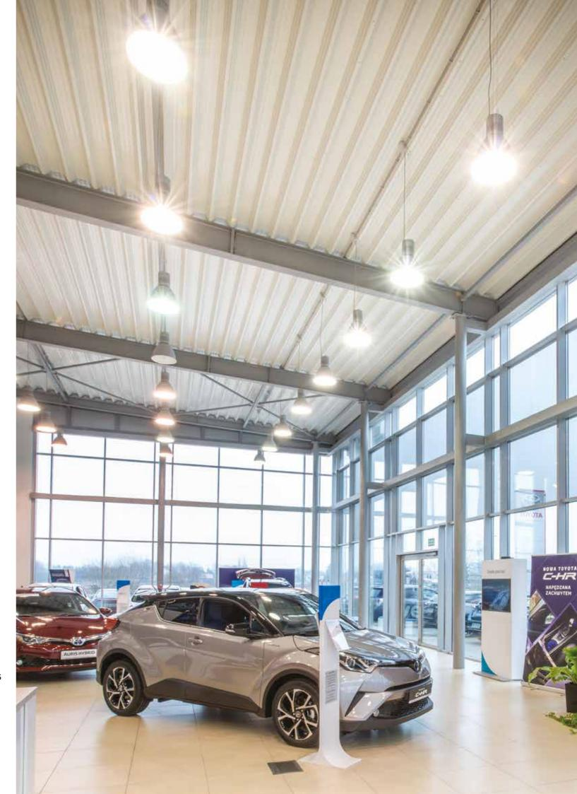
Pendent LED luminaire. Body is made of steel and aluminium and is available in all RAL colours. Light source - Philips, Osram or Tridonic LED module. Standard EVG ballast, DALI or Touch Dali version on request. Acrylic 515 mm reflec or and 1.5 meter suspension set in standard. IP44 cover on request.
